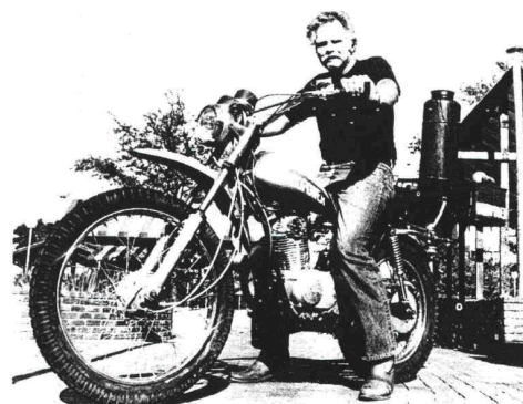
Gainesville, Florida, 1981. The tiny generator that powers this wood-burning motorcycle was constructed at the University of Florida out of a fire-extinguisher casing. The vehicle gets 70 km per kg of wood (20 miles per lb). (Sun Photo by Barbara Hansen)
